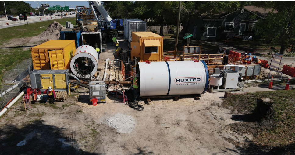
Site setup for 72-in. RCP crossing of I-275 in Tampa, Florida.
